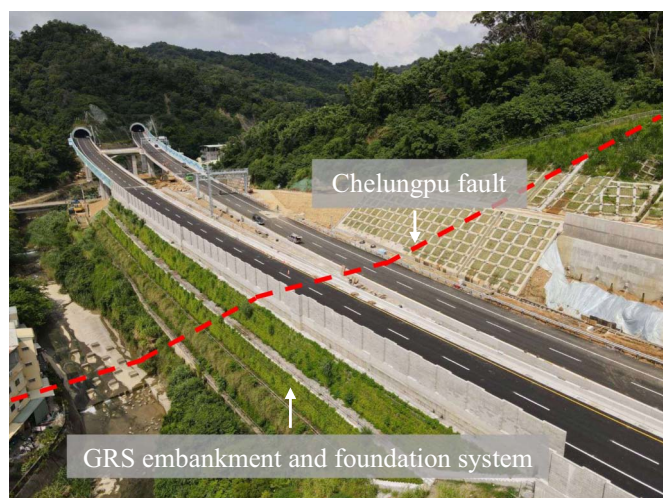
Fig. 1. Reinforced system constructed in central Taiwan to mitigate hazards associated with surface fault rupture. (Image by authors.)
